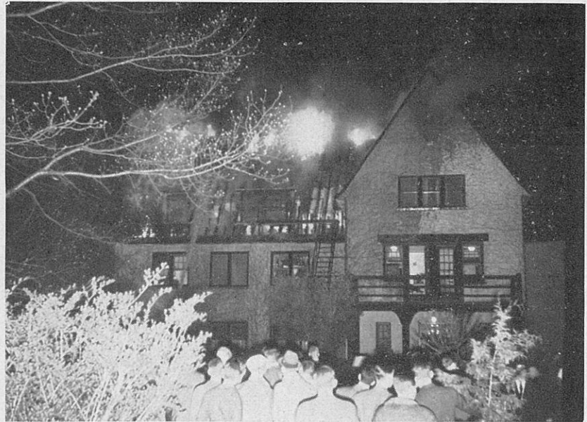
FLAMES WERE SUBDUED considerably when this picture was taken. The shot still gives an idea of the damage, however.
