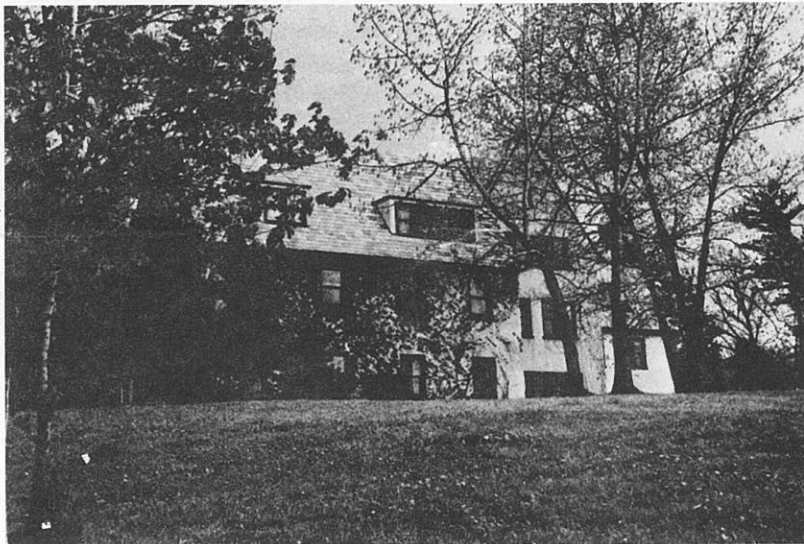
View of the west side of the house.
